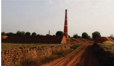
Brick kilns in Kachchh
